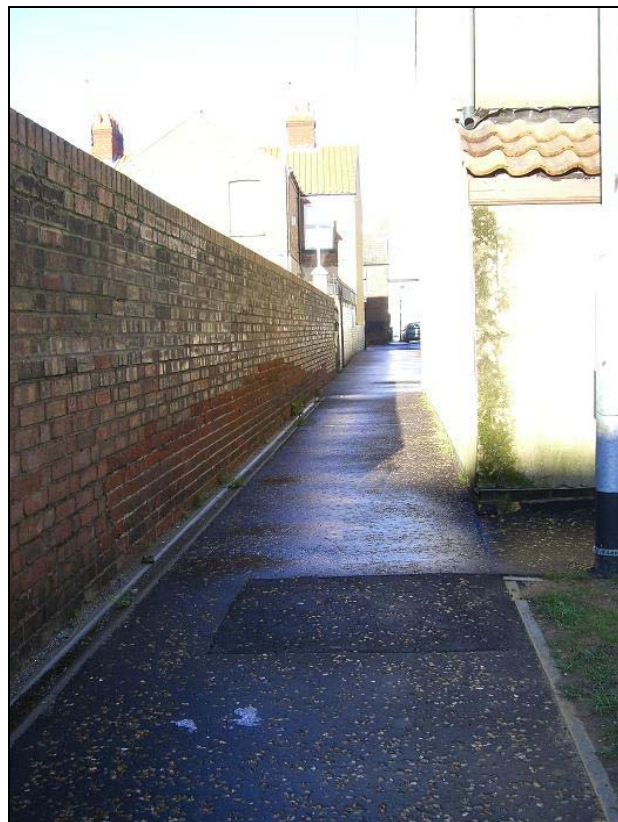
Figure 6: Fox's Passage pavement (January 2009)
