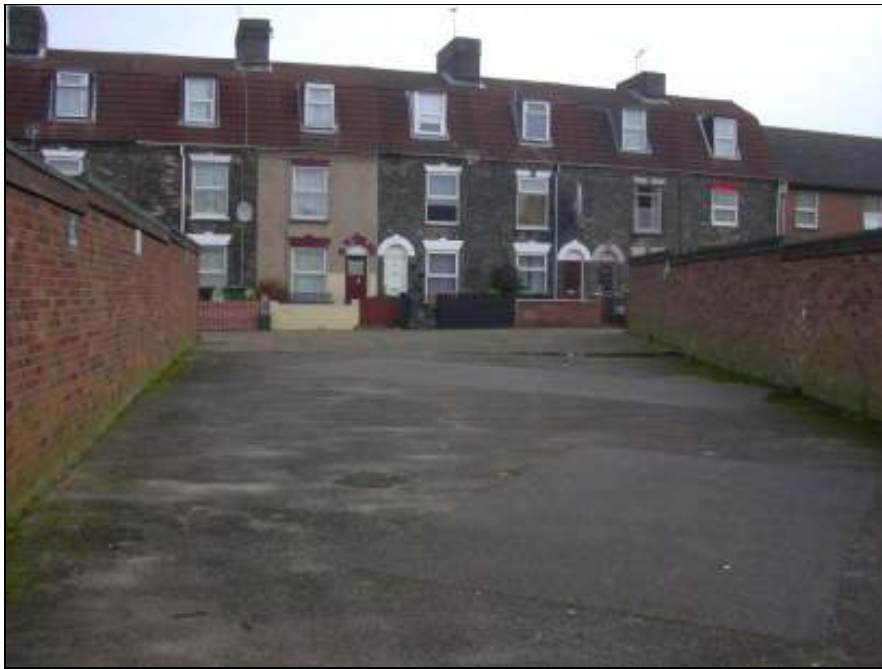
Photograph 5: Shows one part of the area surrounding Swirles Place
